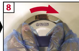
8 Insert new cartridge into housing and turn key to right to lock
