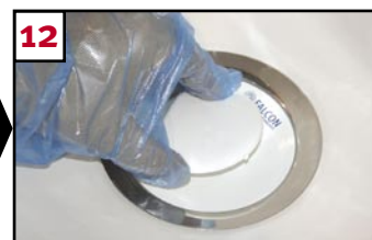
12 Snap the diverter shield into place
