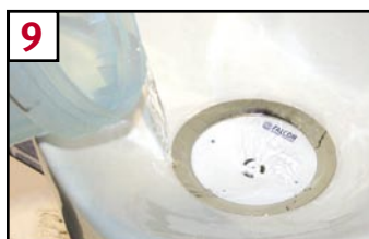
9 With diverter shield removed, fill cartridge with 1 quart or more of water until there are no air bubbles
