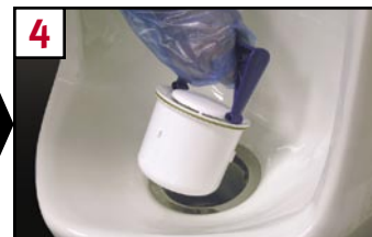
4 Lift cartridge and drain all free liquids
